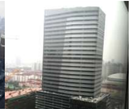
Office Tower 2 - Construction Completed
