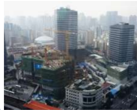
Overall Construction On Track
