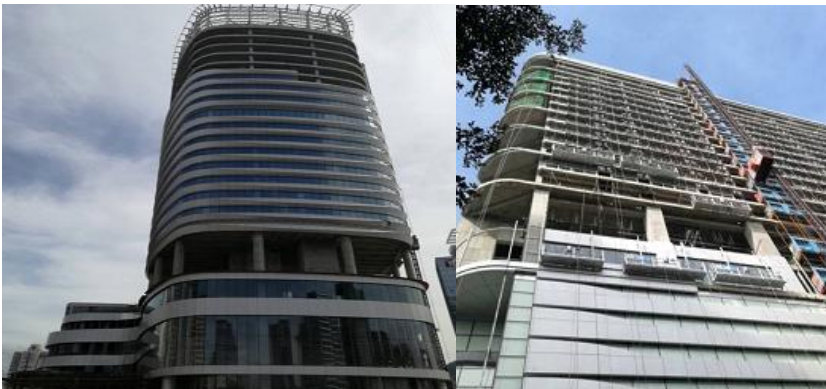
Curtain Wall Installation For Tower Podium
