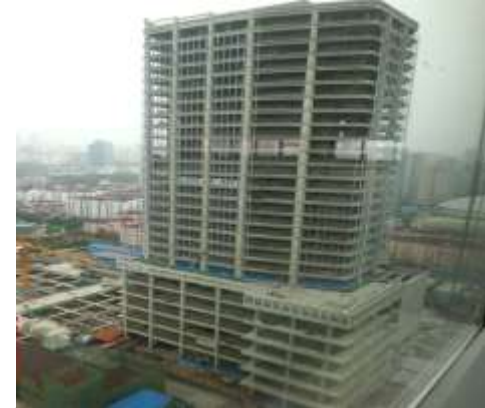
Structural completion for Tower 2
