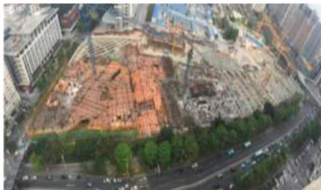
Phase 2: Raffles City Shenzhen Podium built up to level 2
