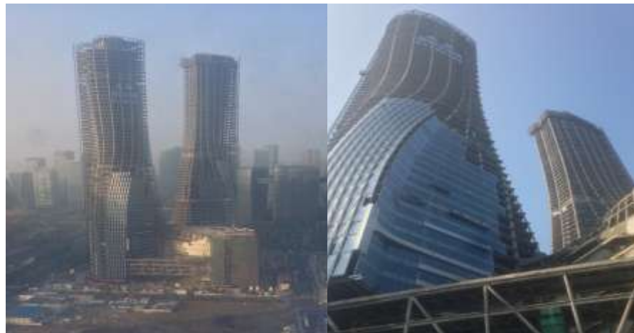
Curtain wall installation in progress
