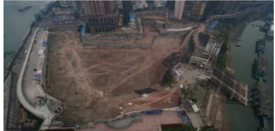
Excavation and lateral support works completed
