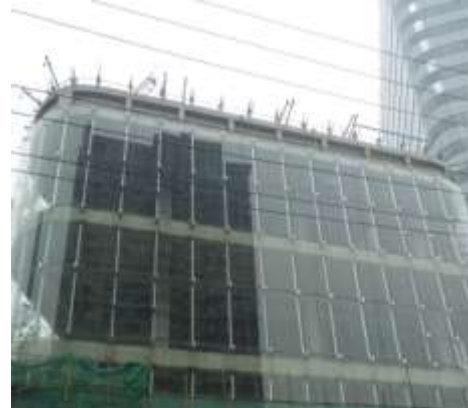
Final stages of curtain wall installation at West Podium and Tower 3
