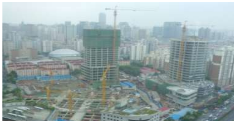
Structural Top-out for Tower 3
