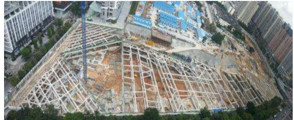
Phase 2: Raffles City Shenzhen Basement construction in progress
