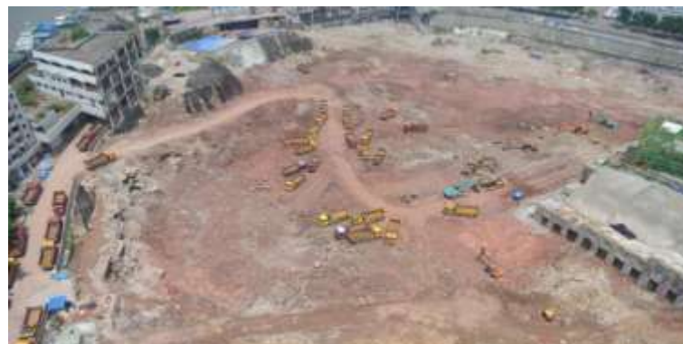
85% of Excavation and Lateral Support works completed
