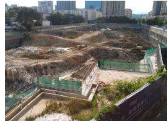
Phase 3: Strata/Trading Excavation in progress
