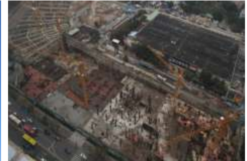
Phase 3: Strata/Trading Basement construction in progress
