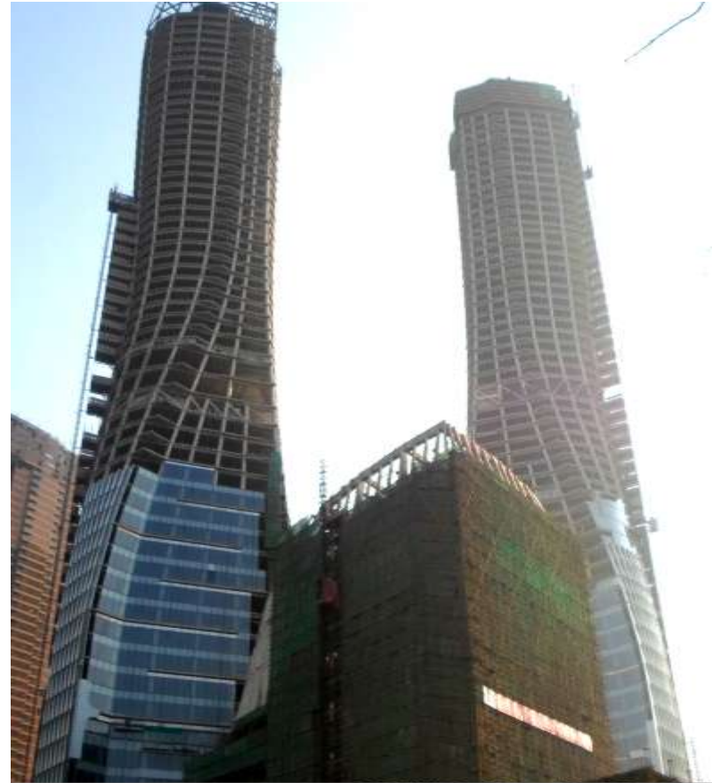
Curtain wall installation in progress
