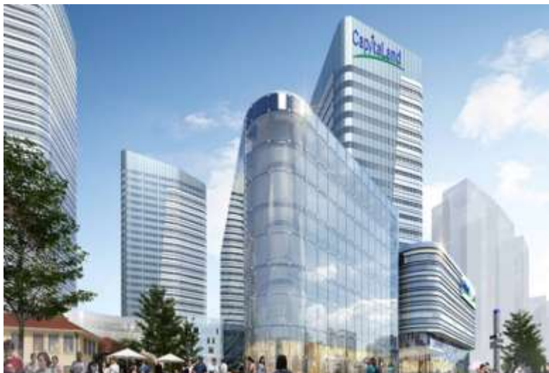
Raffles City Changning Target Opening in phases from 4Q 2015
