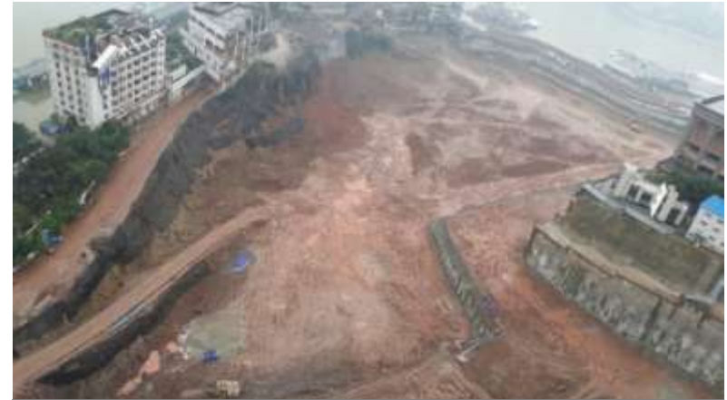
Excavation & lateral shoring works substantially completed
