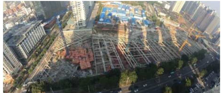
Phase 2: Raffles City Shenzhen Basement construction in progress
