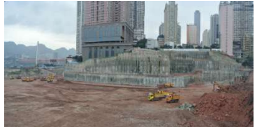
Stepped retaining walls and excavation works substantially completed
