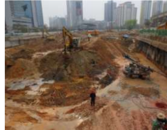
Phase 3 Piling in progress
