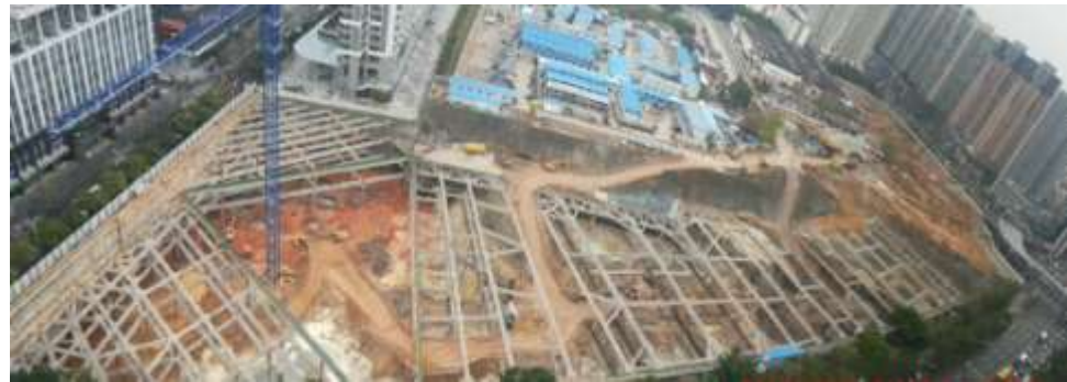
Phase 2: Raffles City Shenzhen Construction on track, excavation in progress
