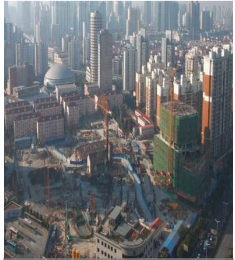
Aerial view: 19% completion
