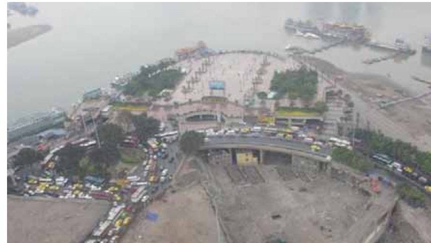
Site clearance in progress
