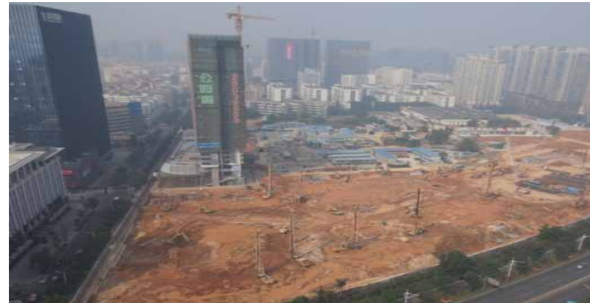
Excavation and shoring system in progress
