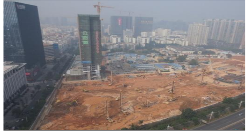
Excavation and shoring system in progress
