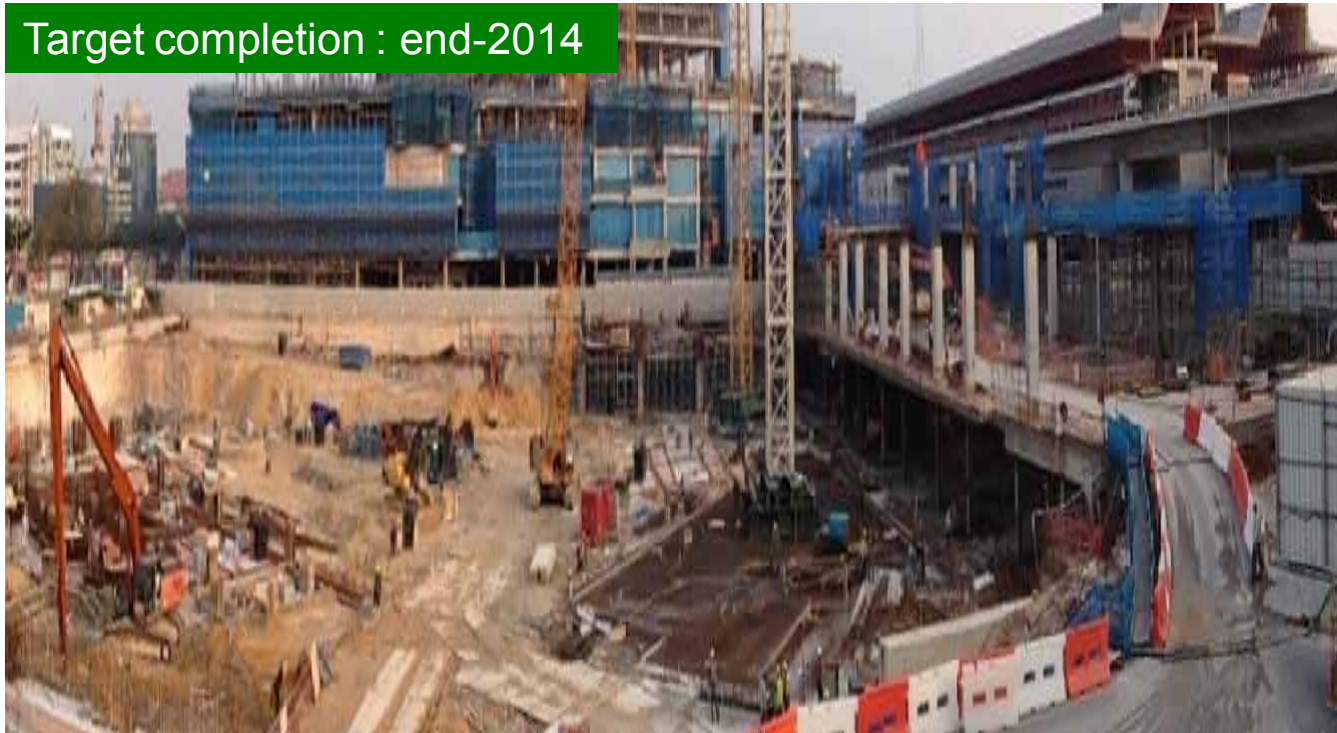
Westgate Tower - Piling Work in Progress
