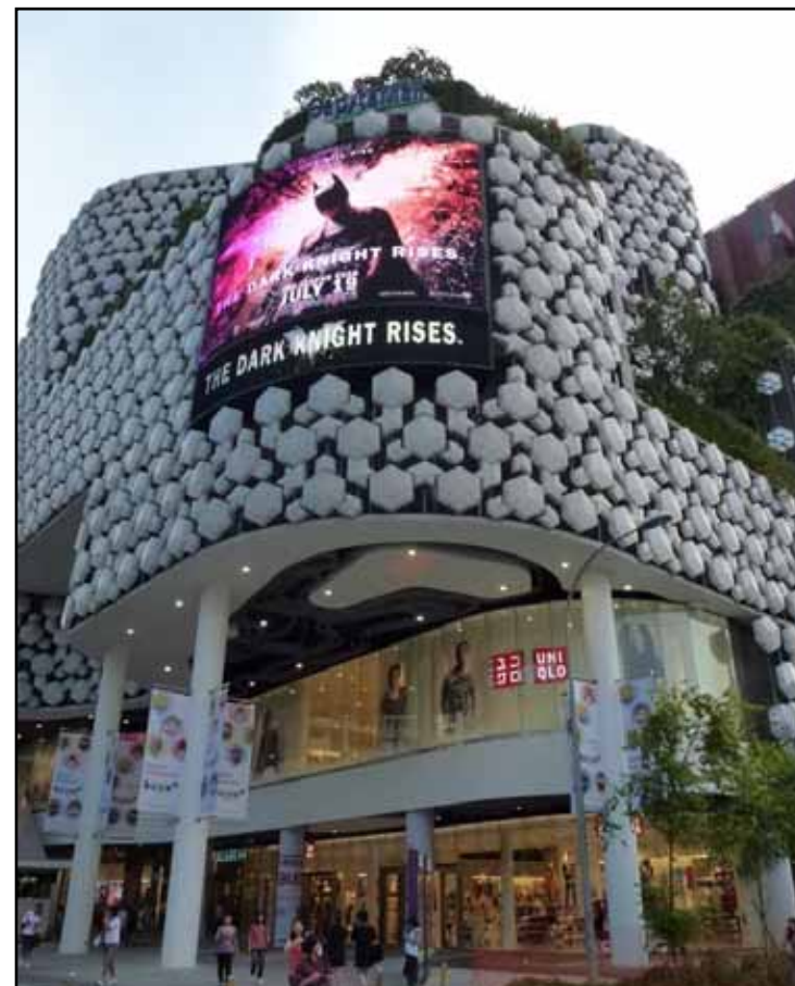
Bugis+'s AEI completed by end-Jul 2012
