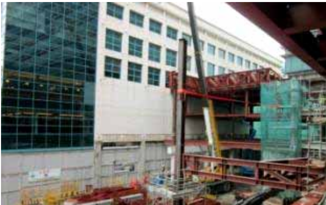
Works on link between Plaza Singapura and The Atrium@Orchard
