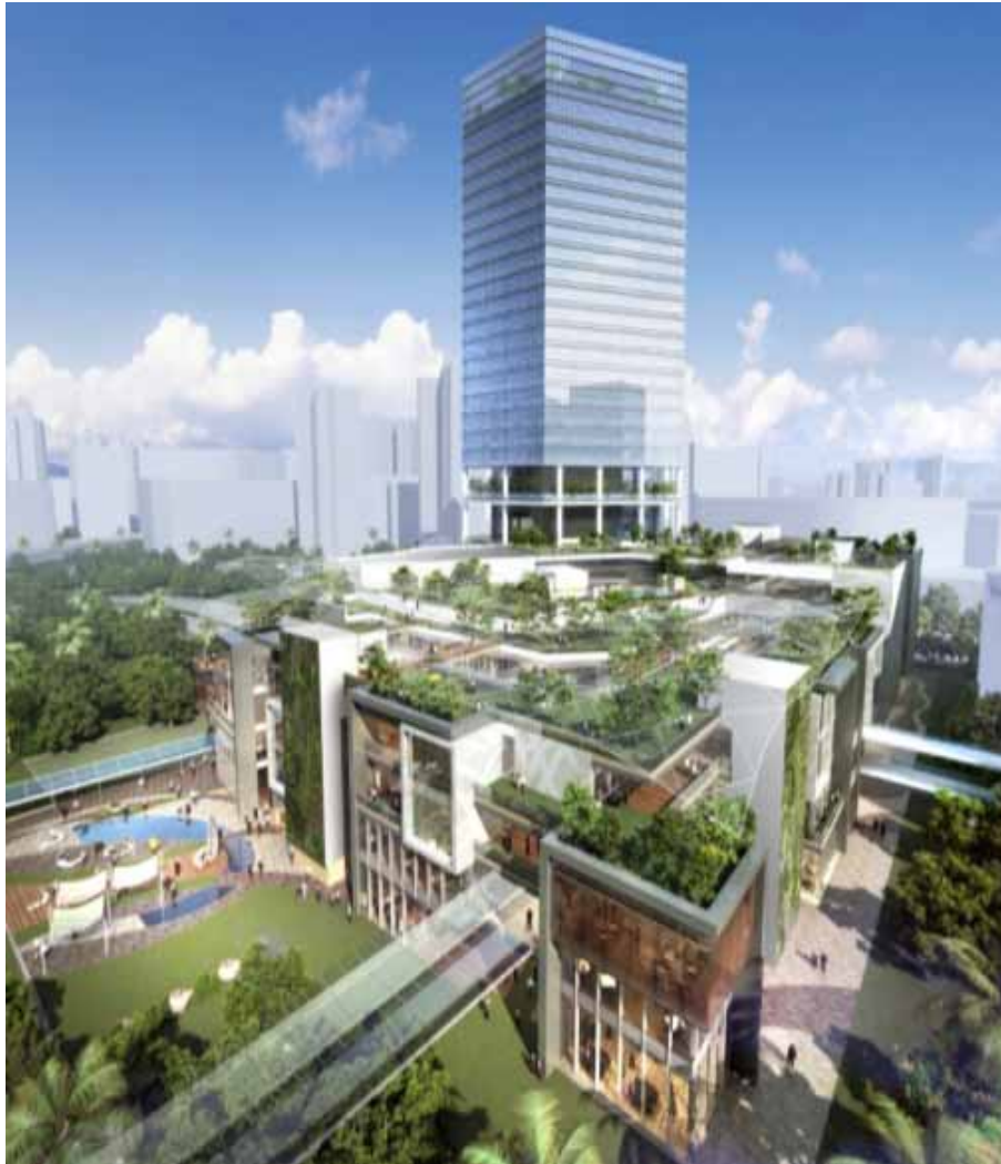
Westgate – New landmark in Jurong Groundbreaking on 12 January 2012
