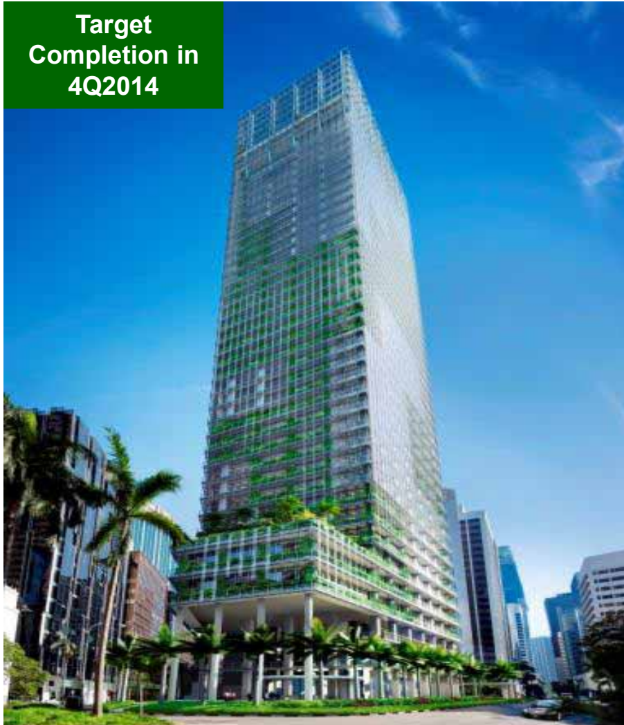
CapitaGreen, a new Grade A office tower Groundbreaking ceremony on 6 February 2012
