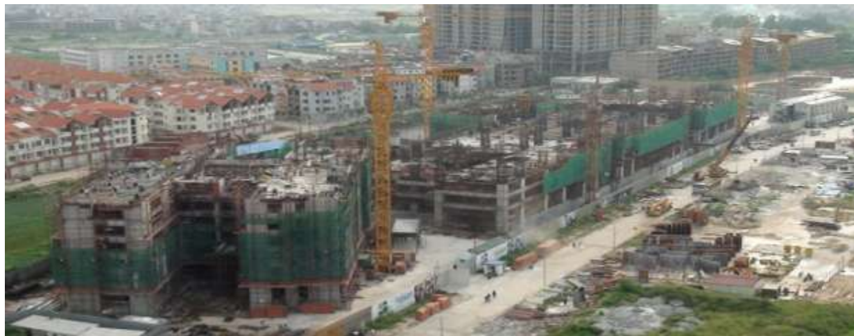
Construction of superstructure in progress
