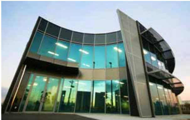
Greens Road, Dandenong, Victoria
