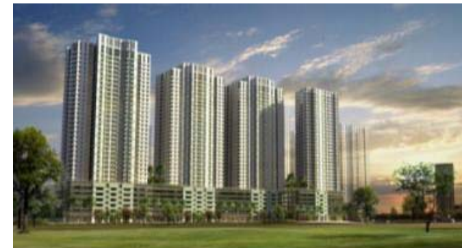
Site at Ha Dong District, Hanoi
