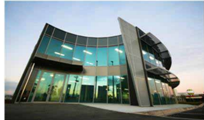
Greens Road, Dandenong, Victoria
