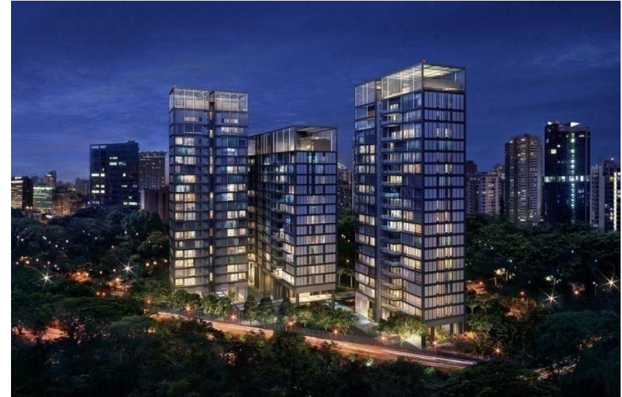
Proposed development at the former Char Yong Gardens site
